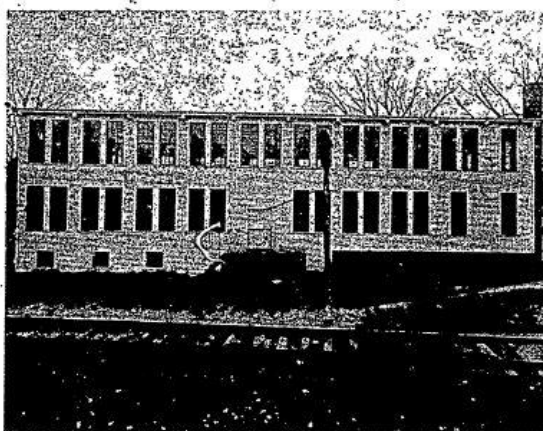
This is the building on Clinton street, Milford, which the Williams & Hussey Machine company will occupy. Another smaller building is not shown in this picture.
